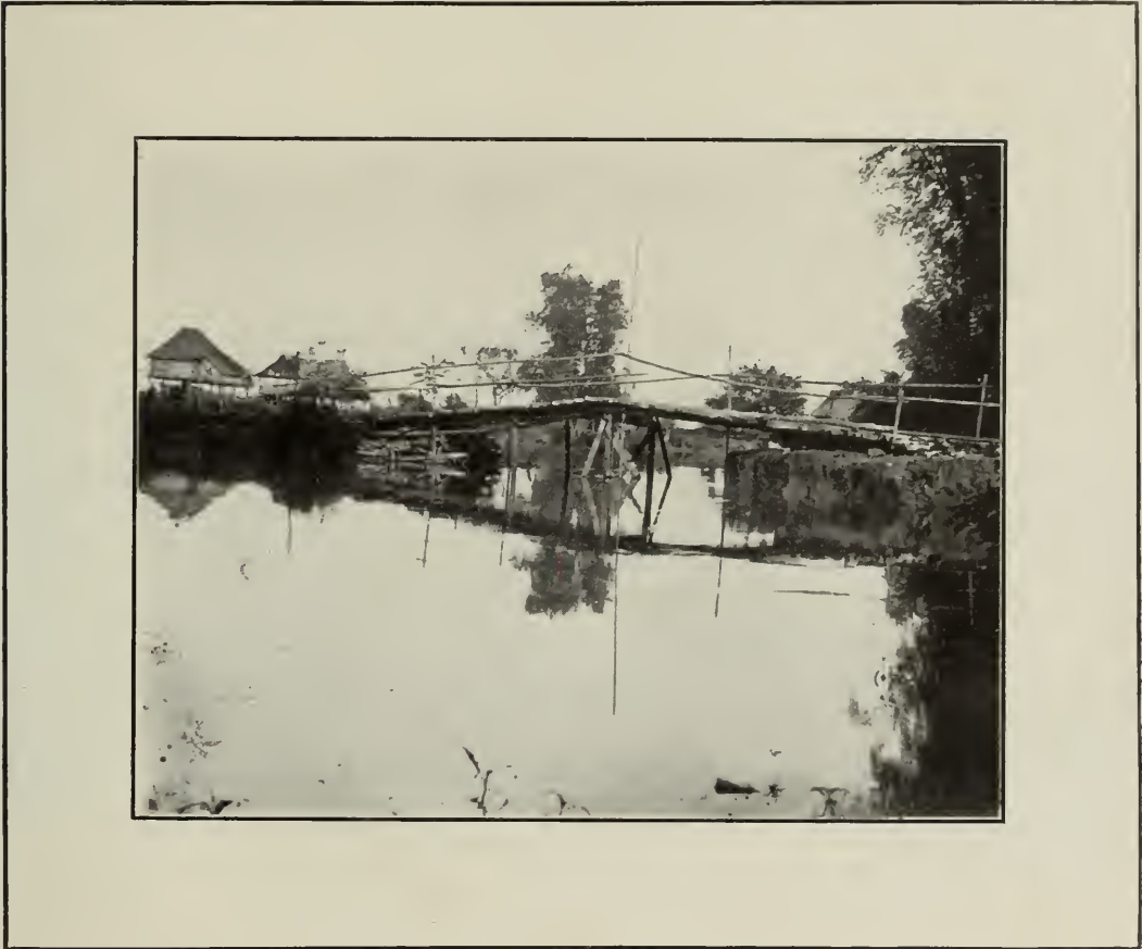
BRIDGE HASTILY ERECTED NEAR CAPAS BY THE ENGINEERS.
